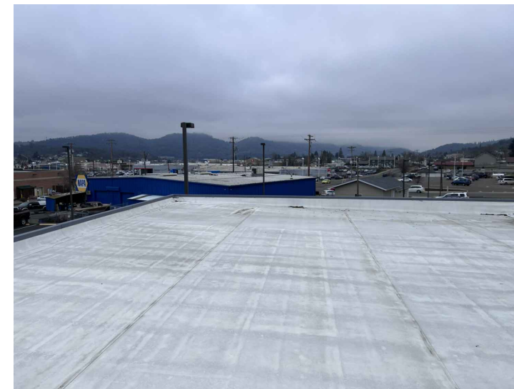
Garage - Roof Area Looking North Existing 4
