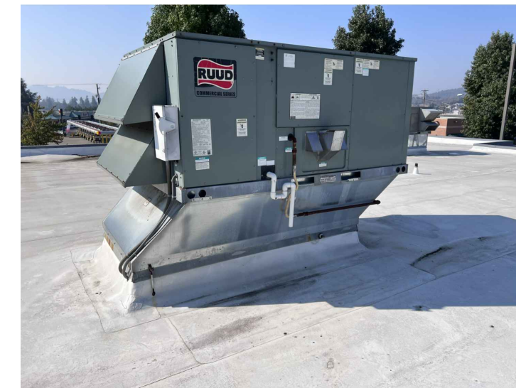
Roof Top Unit Existing 4 NTS
