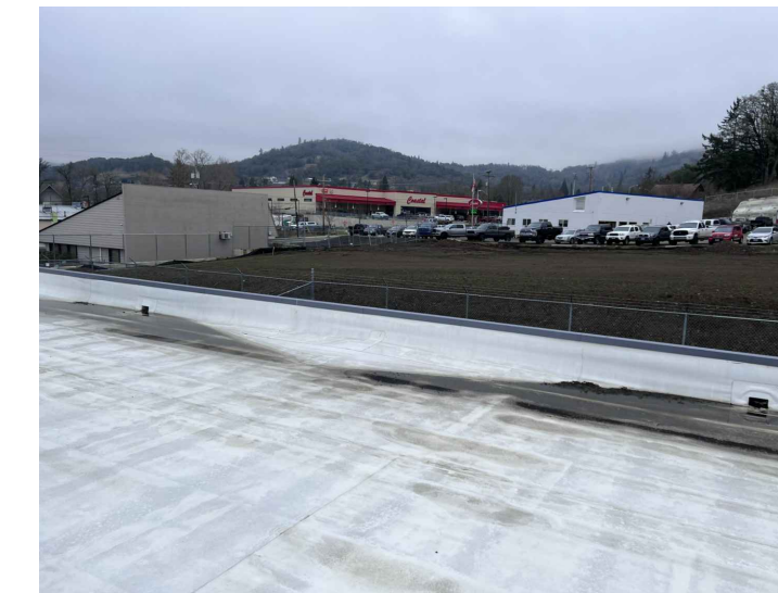
Garage - Roof Area Looking East Existing 1
