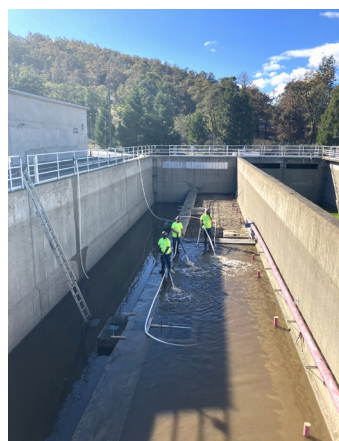
Cleaning and repairs of the Anammox system
