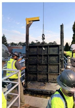
Aeration channel gate removal
