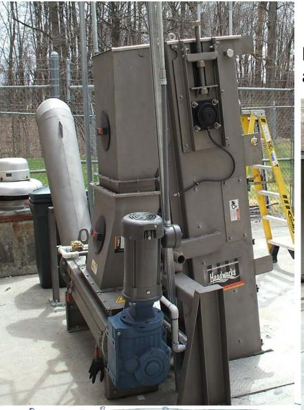
Bar screen with compaction, dewatering, and transport of screenings.....
